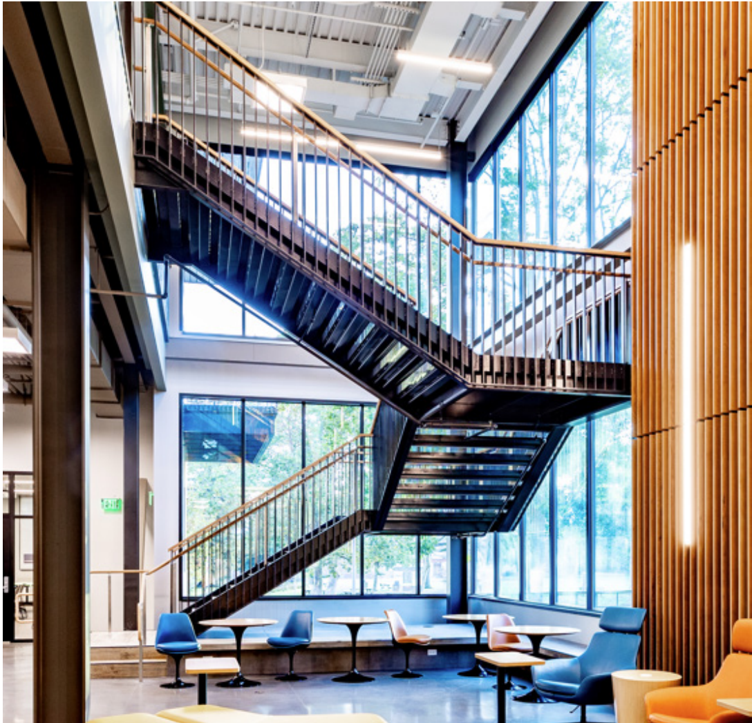
VERTICAL STEEL RODS “NOT RECOMMENDED”
