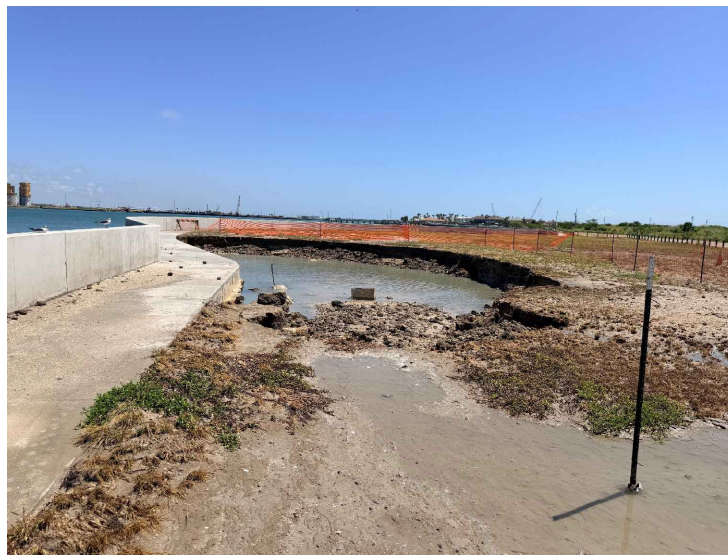
PHOTO 2 - SOIL LOSS BEHIND BULKHEAD FAILURE
